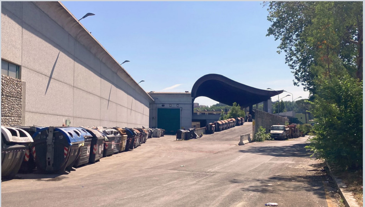
Fig. 1 - TMB Salario was one of the public Mechanical Biological Treatment plants in the city of Rome, required to separate and process undifferentiated waste. The plant received about one-third of Rome's undifferentiated waste: one thousand tons per day (Ama). An estimated four thousand tons of garbage were stationed in the plant daily, the size of a five-meter-high soccer field, only a hundred meters from first homes, 150 meters from a kindergarten (source Internazionale.it, 2018). In use since 2011, the plant, or rather its obvious mismanagement, has catalyzed criticism and protests, generating bitter conflict between residents and institutions, at multiple levels. On December 11, 2018, a fire disabled the plant, to this day still awaiting a convincing and shared redesign
