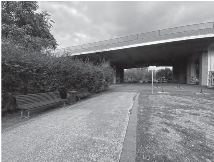
4a-b. The imposing presence of the infrastructure – a permeable threshold between the building fabrics and the public park – mirrored in the water. Photo by the author.
