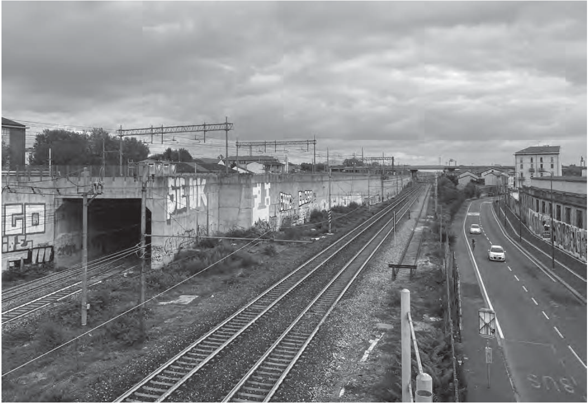
2. The complex of infrastructural lines from the city towards the Segrate railyard between via Tucidide and via Camillo and Otto Cima. The section is made by a sequence of many types of infrastructures – sidewalk, road, 10 rails placed on several levels, sidewalk, road, sidewalk, cycle path – with the A51 Tangenziale est in the background. Photo by the author.
