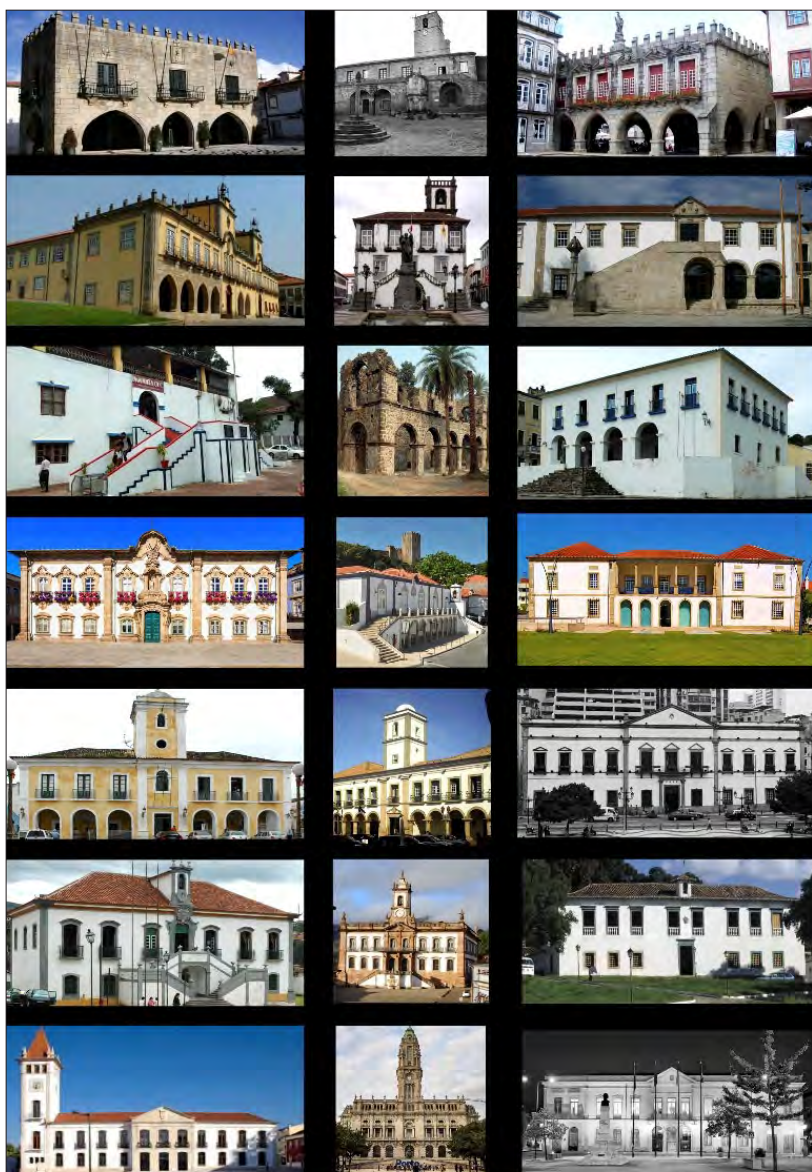
Fig. 4 – Casas da Câmara (Source: photograph by the author)
