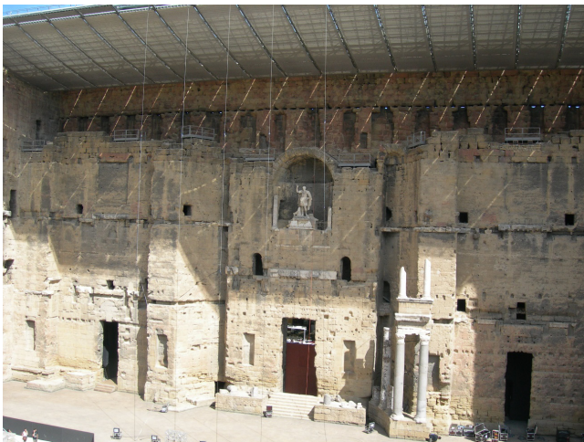
Fig. 1 – The stage front of the theatre in Orange with the new roof to contain all the installations necessary for cultural performances
